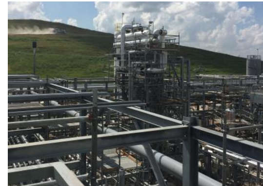
Monetisation of landfill gas
