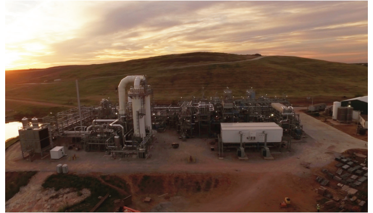
Envia plant showing the SMR tower on the left with FT island behind it on the right side
